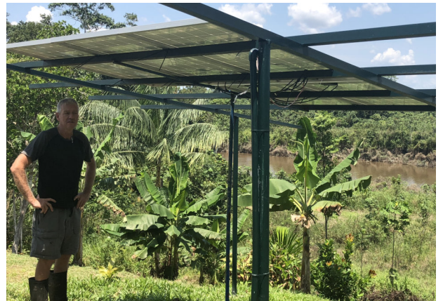
Devon Graham, Director of Project Amazonas, standing under the solar panels used to generate electricity to power the system
